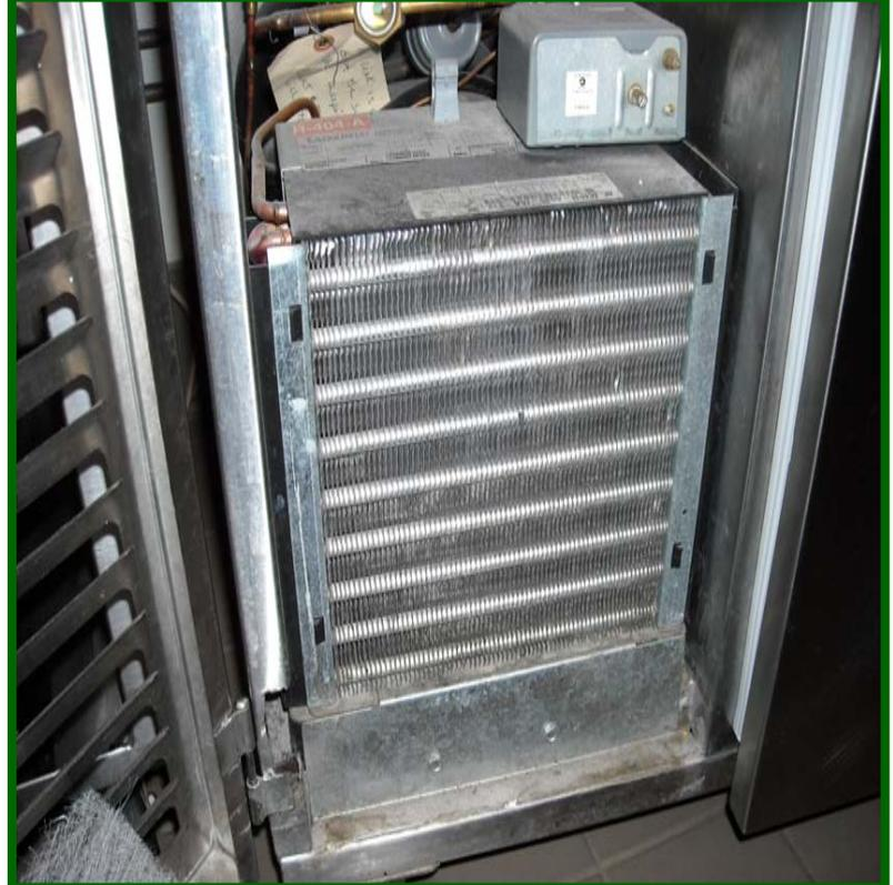
The unit in this picture is on a 60-day Preventative Maintenance (PM) cycle....Notice how clean the fins and tubing are in this picture
